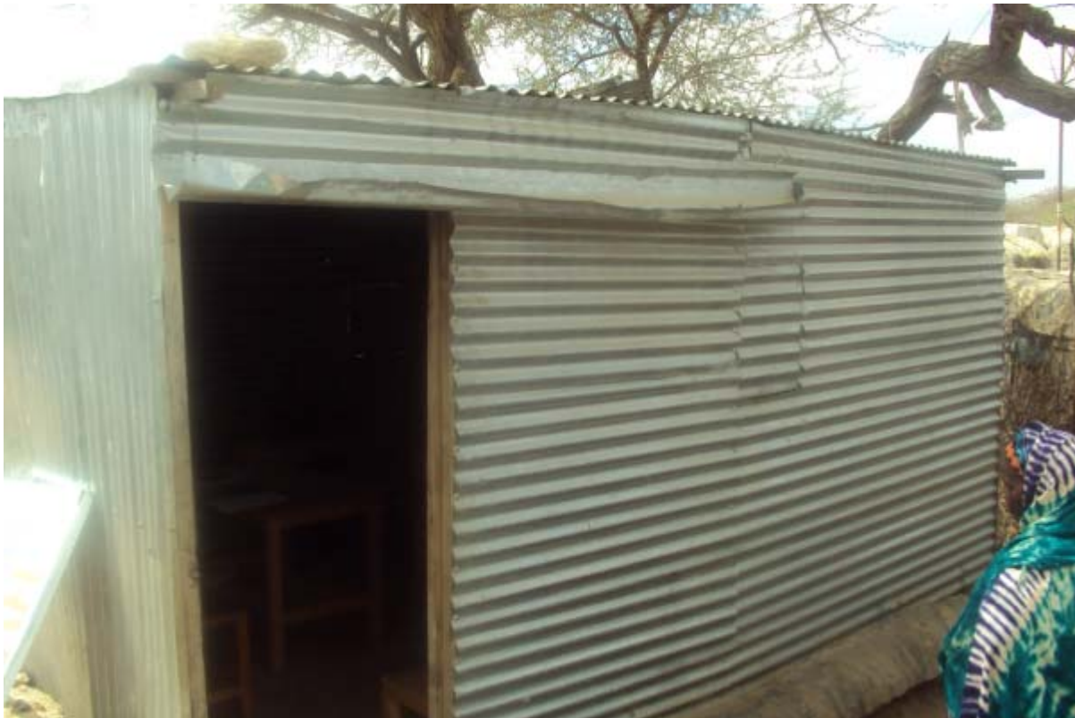
Picture 8: This community structure measuring 3x3 metres is what accommodates 30 students. Some camps like Berbera do not even boast of such facilities.
